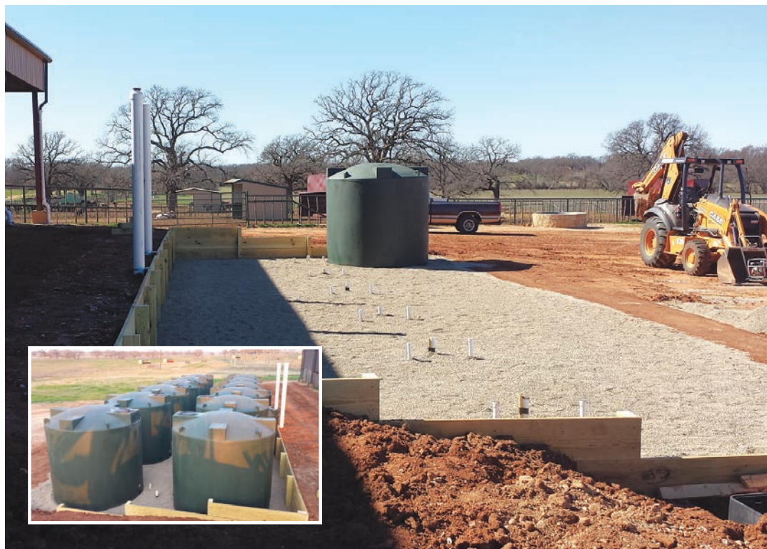
A rainwater collection system can be customized so as not to disrupt the aesthetic appeal of a facility. Circle Y's largest system was built on a pad site approximately 3 feet below ground level, with a retaining wall used to protect the unit.
